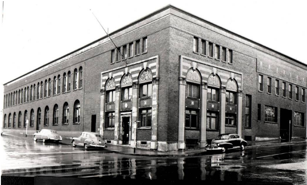
Yale Union Laundry Building, circa 1950 OHS Negative # CN 006589 Photograph to be used for reference use only
